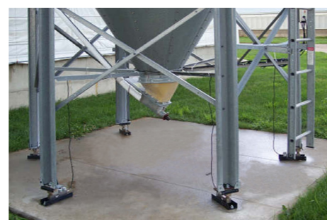
Load Cells handle up to 10,000 pounds (4,500 kg) per feed bin leg.
