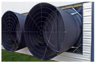
Chore-Time's 57-inch EnduraMax™ Direct-Drive Fan with HYFLO® Shutters features a variable speed motor to help maximize energy efficiency.
