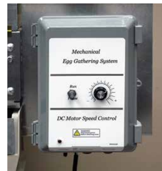
Egg flow to the table is controlled by a run/pause toggle switch and a belt speed adjustment knob.
