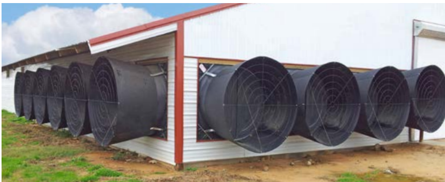
Chore-Time's Energy-Efficient, Corrosion-Resistant 57-Inch (145-cm) ENDURA® Fans
